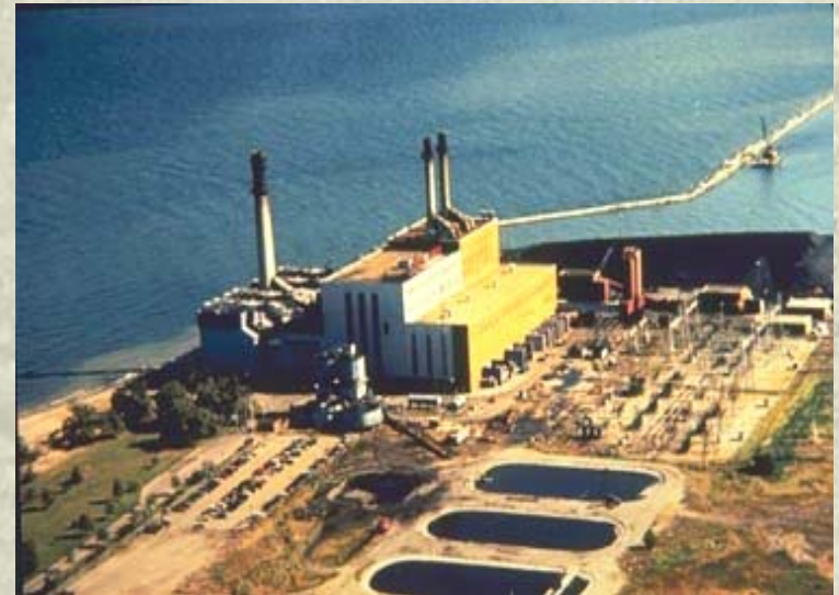
NRG Dunkirk power plant on Lake Erie
